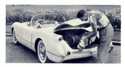
THE SLEEK REAR DECK of the Corvette conceals a generous luggage compartment—far more spacious than most sports cars. The spare tire is in a well under the floor; the radio antenna is built into the deck lid.
