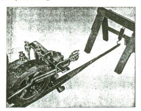
Buick Motor on testing stand, with Brake on the fly-wheel, in making the December 22, 1904, test, in which the Buick Motor, a pair of opposed 41/2 x5!nch stroke cylinders, showed better than 29 BRAKE HORSE POWER at 1320 crankshaft turns per minute.
